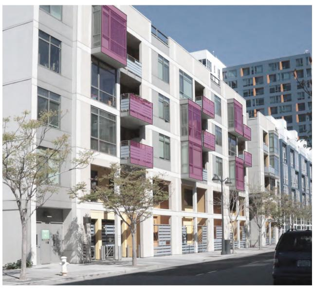
Above is an example of how to calculate the encroachment area with a variety of bays and balconies, demonstrating both enclosed and unenclosed encroachments. Shaded faces would be included in encroachment area calculation. PHOTO: PERKINS+WILL
