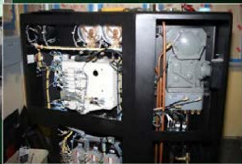
Additional work is being done on the low-volt wiring system, connecting components to the electrical cabinet.
