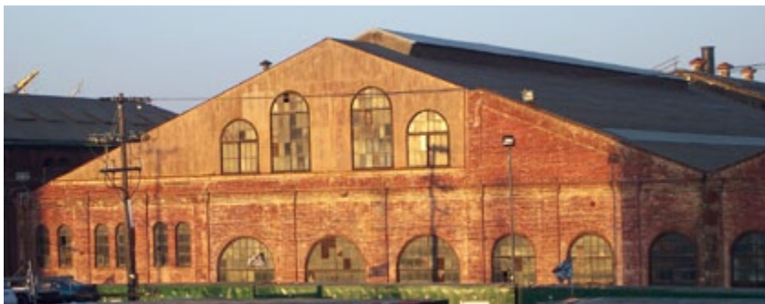
Union Irons Works (Building 113/114) - Photo Ralph Wilson
