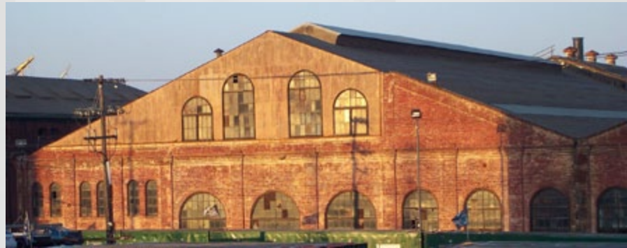
West Façade of Building 113, 2004 (Photo: Ralph Wilson)
