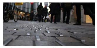
Aural/'noise' paving: integrated 'rumble strips' provide an aural warning cue for approaching traffic at intersections and turns. NO SOURCE FOUND
