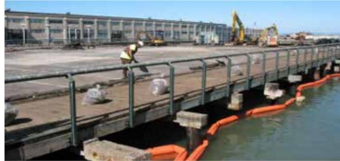
Floating boom is deployed around construction work to capture debris.
