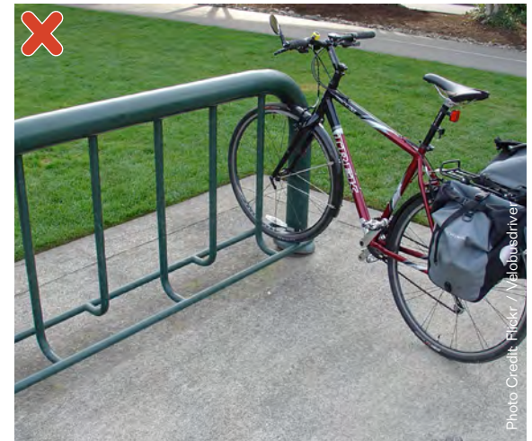
Rack design does not allow for bicycles to be properly secured
