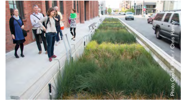
Sidewalk with Stormwater Planter
