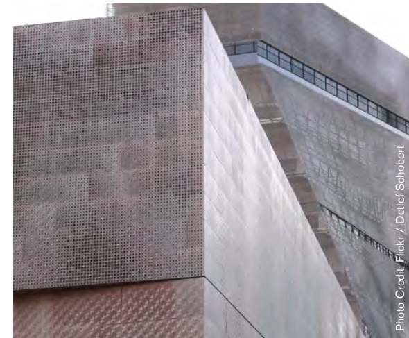
Treated Perforated Metal Panels Intended to Patina (Exemplary Performance – Materiality) DeYoung Museum, San Francisco
