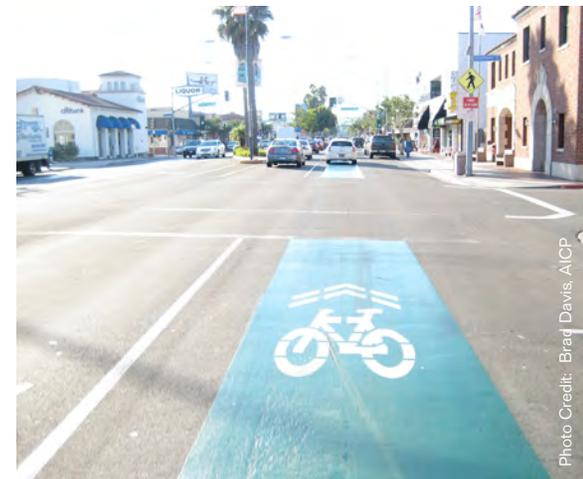
**FIGURE 4.5.3:** Example Class 3 Shared Lane (Super Sharrows) Pavement Marking
