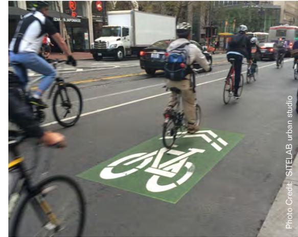
**FIGURE 4.5.2:** Example Class 3 Shared Lane (Sharrows) Pavement Marking
