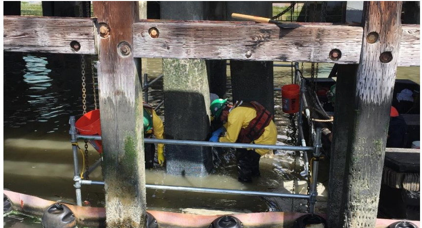
Working at low tide to strengthen wharf decks and piers © SGH
