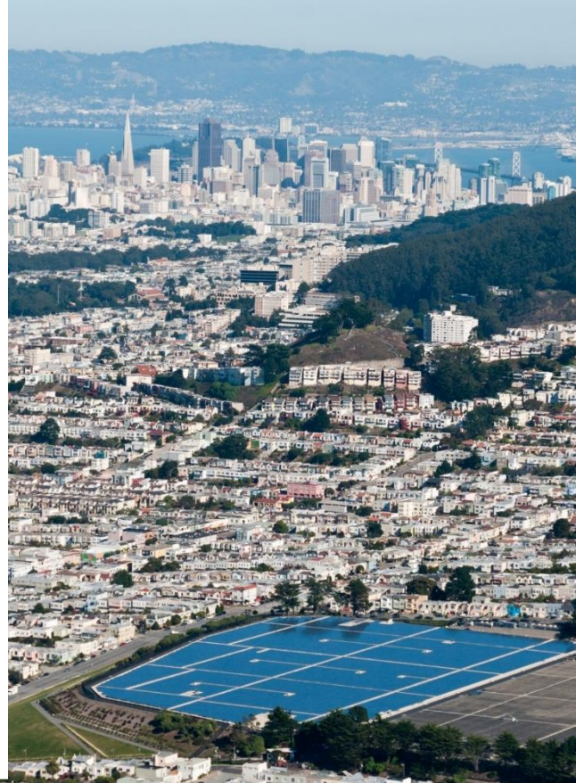
Solar Panels at Sunset Reservoir
