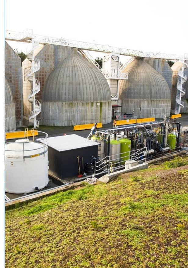
Oceanside Treatment Plant
