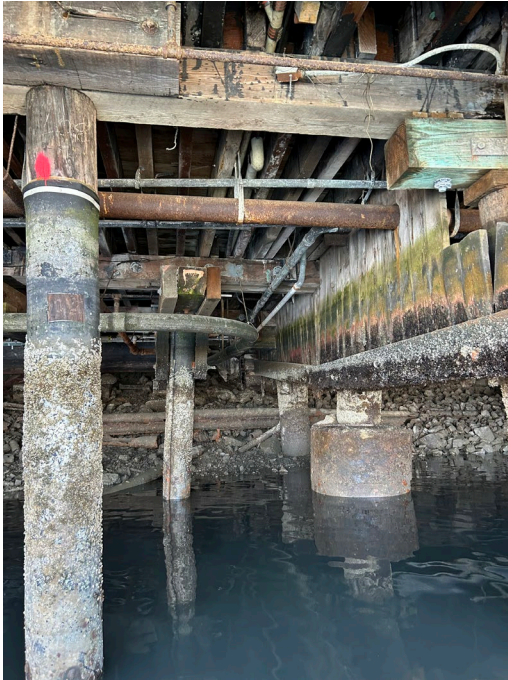
Existing firestop wall:
