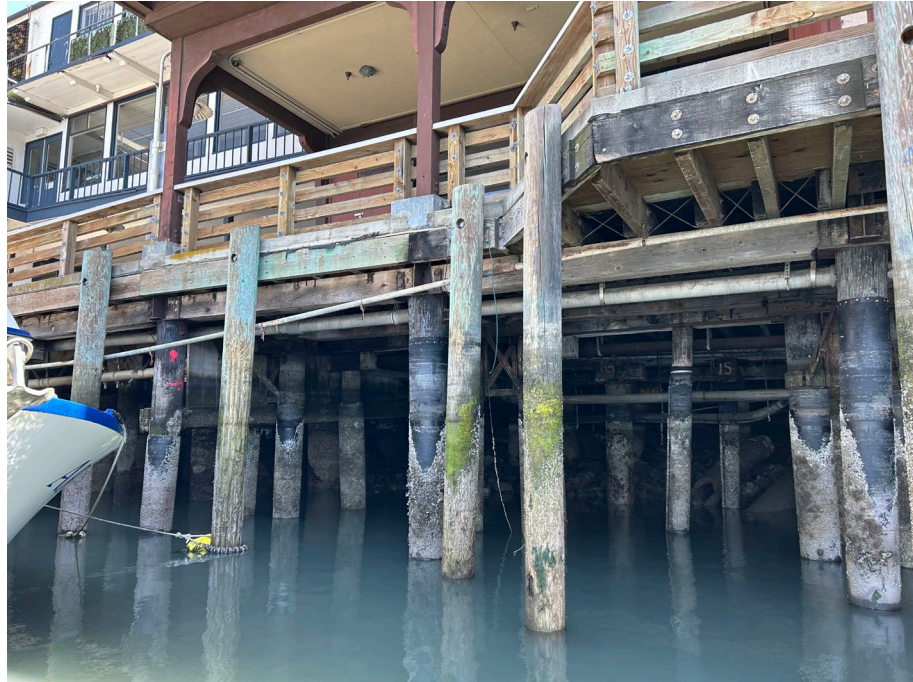
Existing timber piles:
