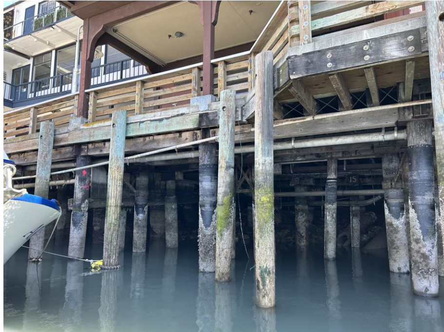
Existing timber piles:
