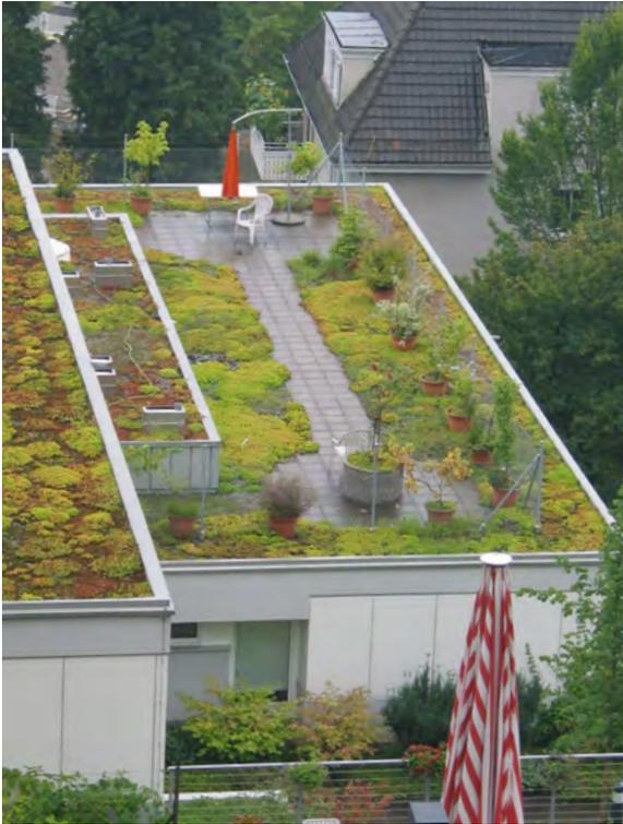
*Intensive vegetated roofs can provide usable open space in addition to their stormwater management function. Photo: Rosey Jencks*
