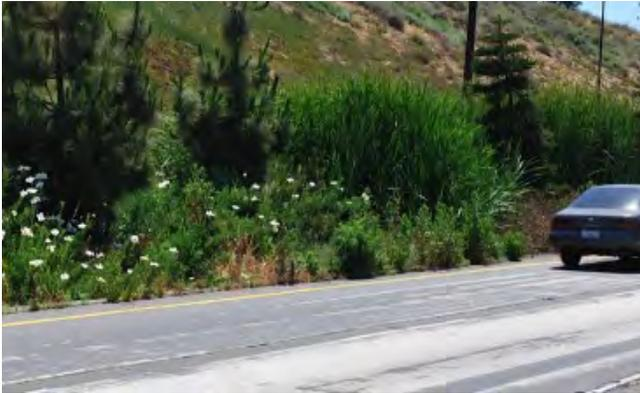
*This vegetated buffer strip along the Imperial Highway in Los Angeles, CA slows stormwater runoff from the highway.
